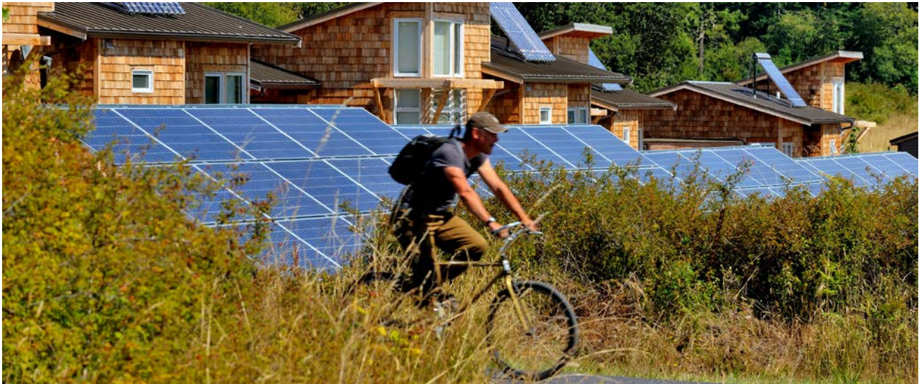
Solar panels at Common Ground, an LEC project by Lopez Community Land Trust (Lopez Island, WA)
